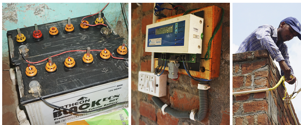
Figure 4.3. Vulnerable pico-grid system units (from left to right): Battery bank was subject to power theft; Energy meters were prone to technical failures and tampering; Distribution system connection points sometimes had to be repaired after an accidental interaction with a passer-by (e.g. a vehicle or a human). Photos: Sini Numminen 2016
