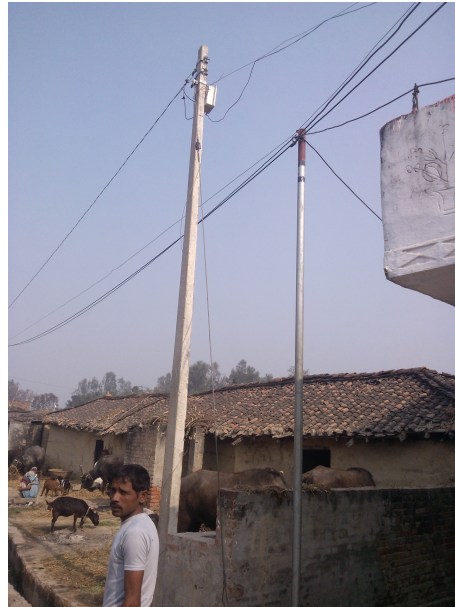
Figure 5.1. A single village may be served by both a government distribution system (concrete pole, on the left) and a micro-grid system (steel pole, on the right). Photo: Sini Numminen, 2018
