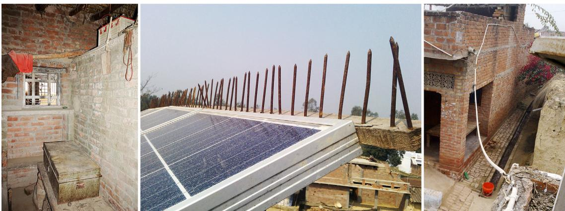
**Fig. 2.** a–c (from left to right). Placing of a central battery bank up on the loft of a storehouse (a); Technician attached a row of nails on top of the PV panel to prevent birds from landing there as bird leaves, dirt and shadowing reduce the solar energy output (b); Faulty cable installation dangling over a village alley (c). Photos: Sini Numminen, 2016–2018, various micro-grid sites.
