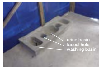
... faeces and urine are separated through the Eco-san interface here...
