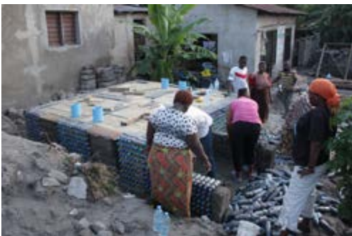
During phase two, PU building the “Pilot Toilet” base with recycled bottles.
