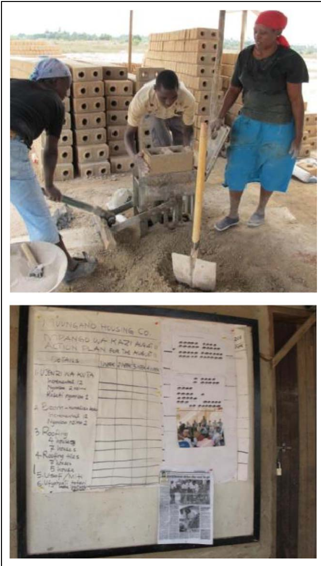
Figure 5. Chamazi housing construction: On-site interlocking bricks and action plans.
