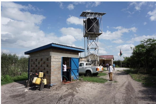
1st generation of Grundfos Lifelink water ATM, and a complete water kiosk Photo credit @
