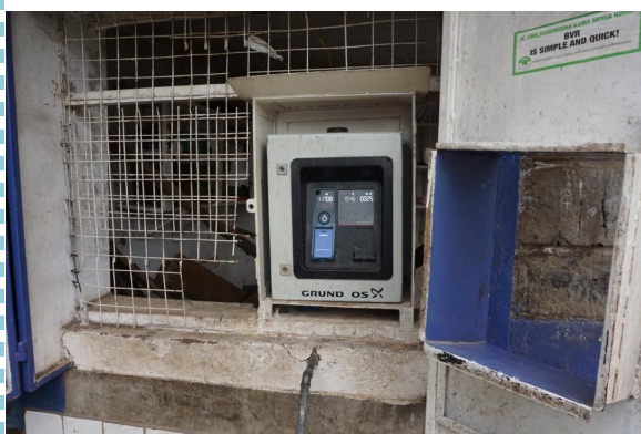
3rd generation of Grundfos Lifelink water ATM, commercialized as AQtap. Photo credit @
